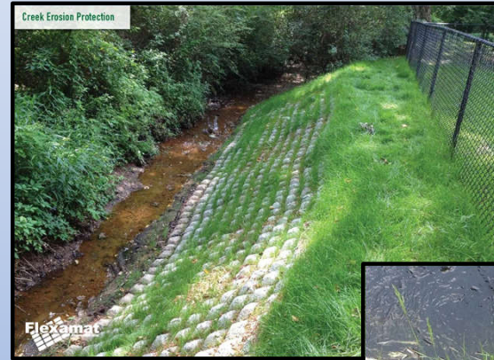
Flexamat Bank Stabilization
