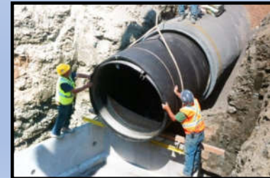
Inline Tideflex Valve M Street and L Street Outfalls
