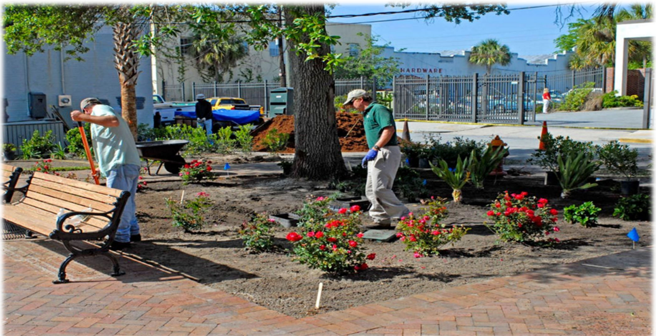
Jekyll Square West Under Construction
