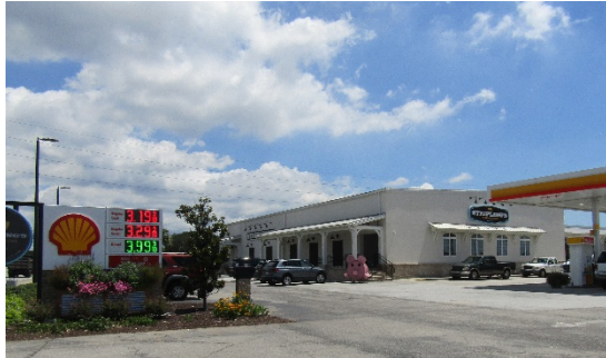
Re-purposed auto dealership building for a Striplings General Store on Glynn Ave.
